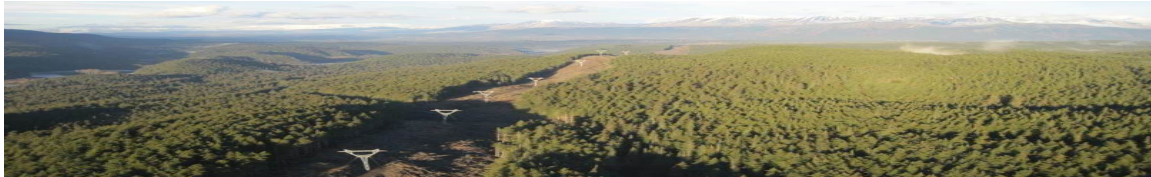
BC Hydro NW Transmission Line Photo credit: Valard LP
