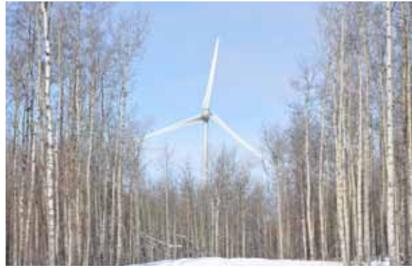
Wind turbine at Bear Mountain Wind Farm, Dawson Creek, BC.
