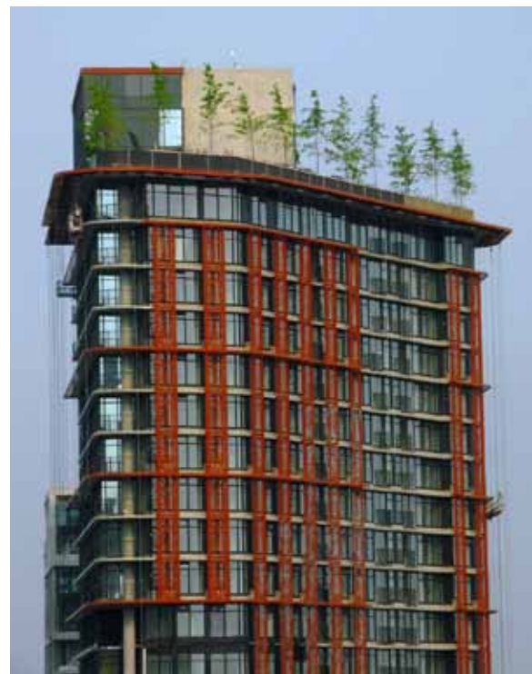
Green roof on Vancouver high-rise.
