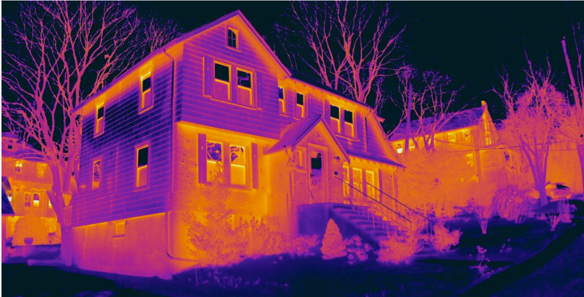
Figure 1: A thermal image of the front façade of a single family home © Courtesy of Essess, Inc. http://www.essess.com/technology/machine-vision/
